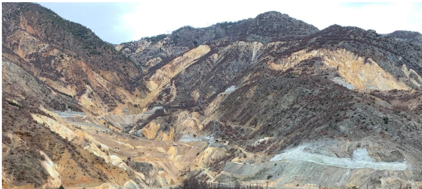
Figure 5. Start of initial earthworks at the Hod Maden site, March 10, 2023.
